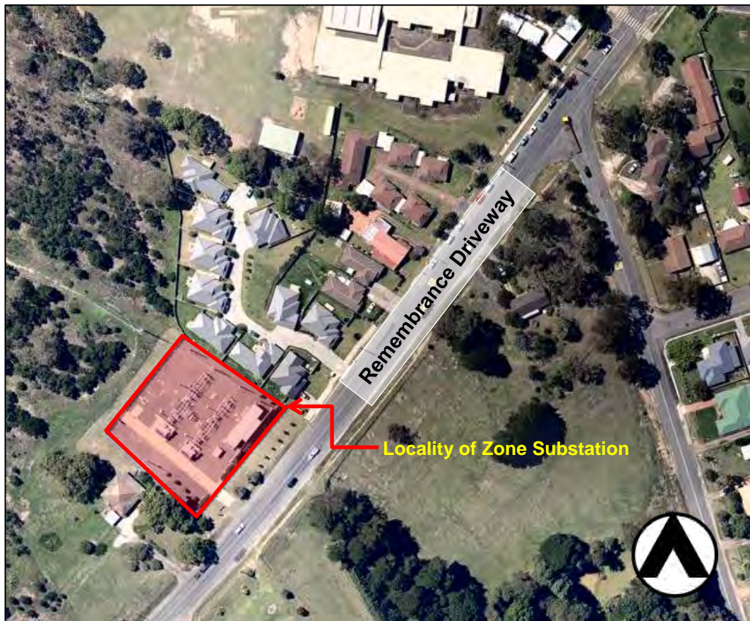
Figure 2 Tahmoor Zone Substation (Image source: NearMap)
